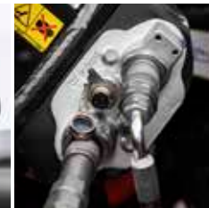
Built-in electric socket (2 lines)
