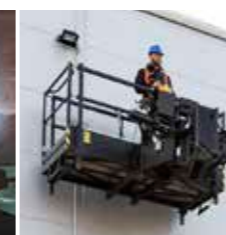
Man platform ready
